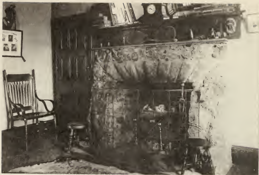
Figure 59. Smoking room fireplace installed by William Henry Wetherill, 1890s or early twentieth century. The wood lintel and mantel for the original large cooking fireplace opening is visible above the river stone surround. (Mill Grove Files, Audubon, PA)
